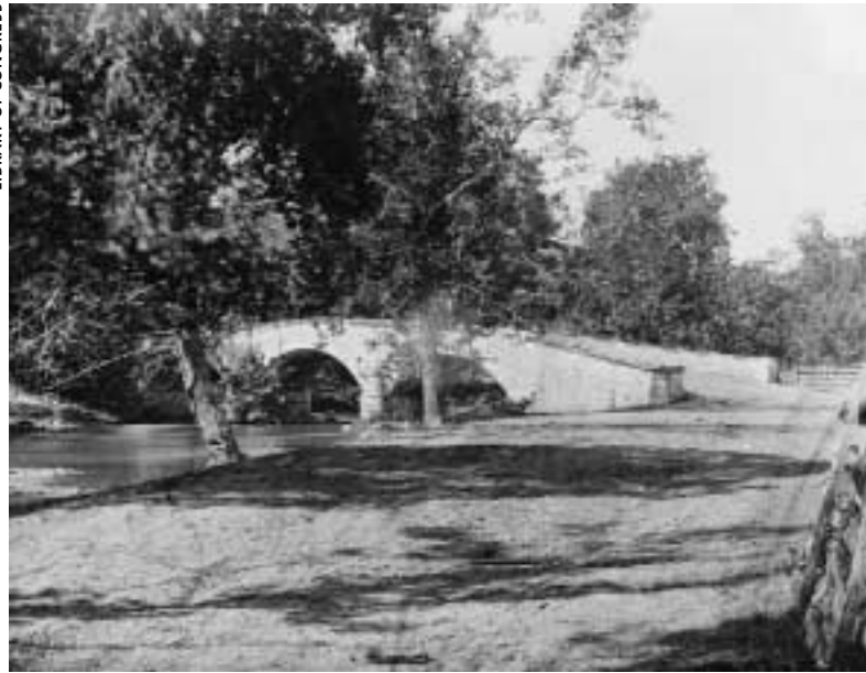
Burnside's Bridge was a peaceful place in this 1880s photograph.
